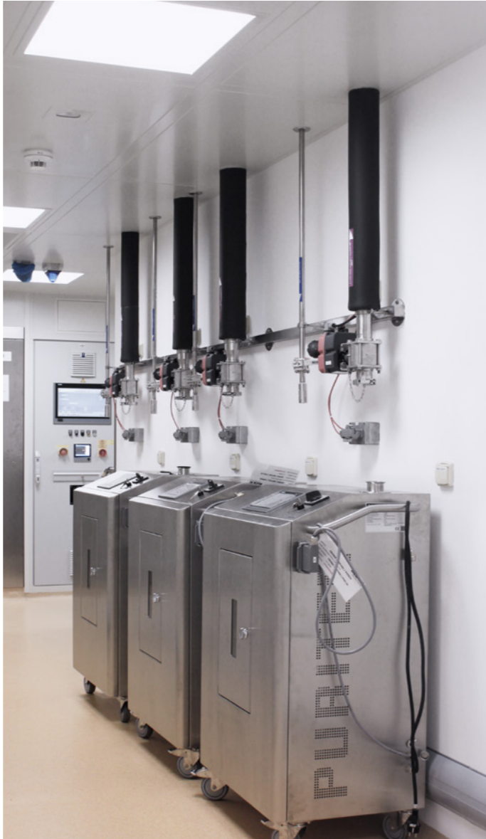
Mobile Hydrogen Peroxide Vapour Generator – Puriter, Praha Vaccines a.s. / NOVAVAX CZ a.s., Czechia
