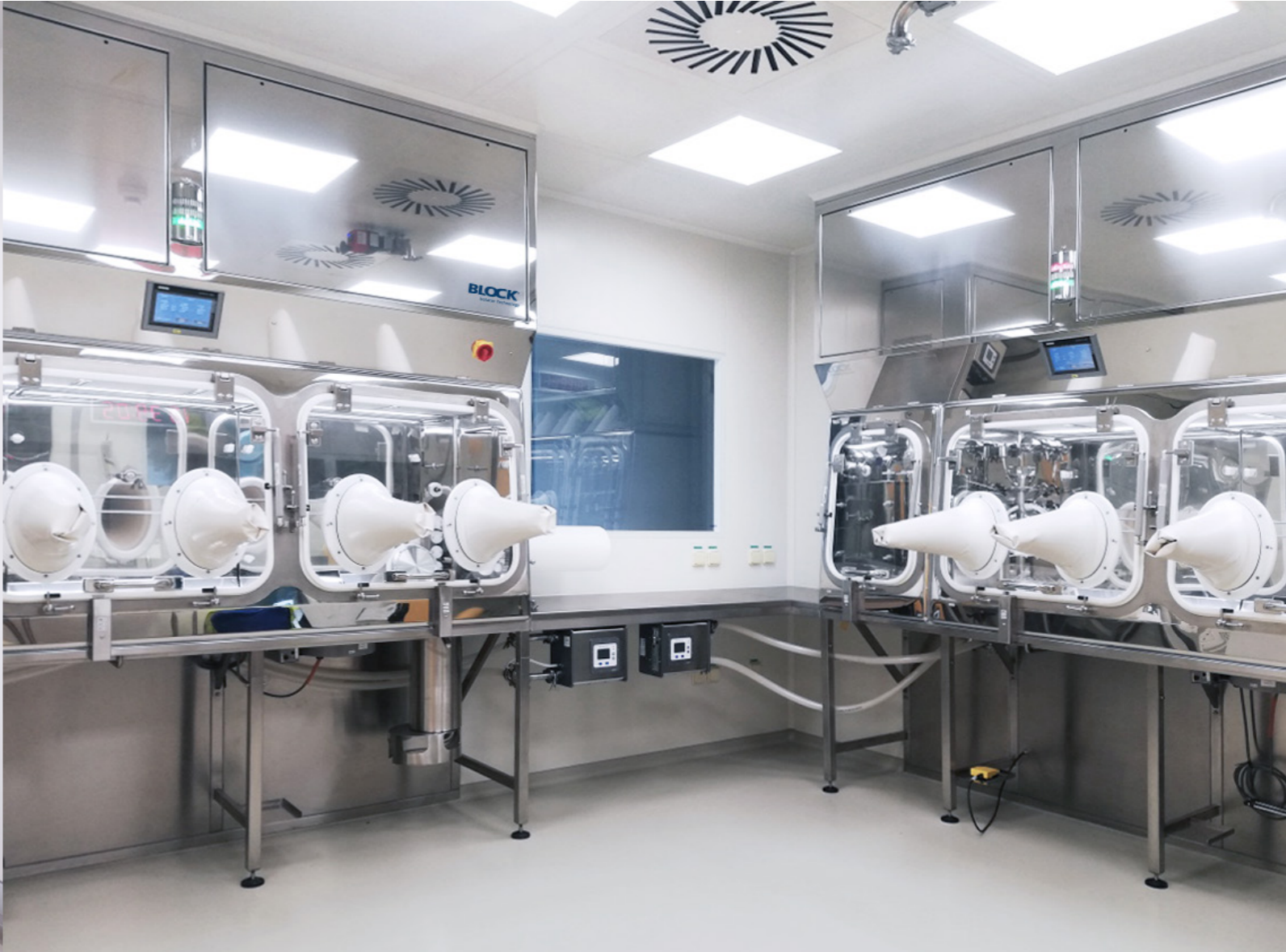
Isolator for product protection, Praha Vaccines a.s. / NOVAVAX CZ a.s., Czechia
